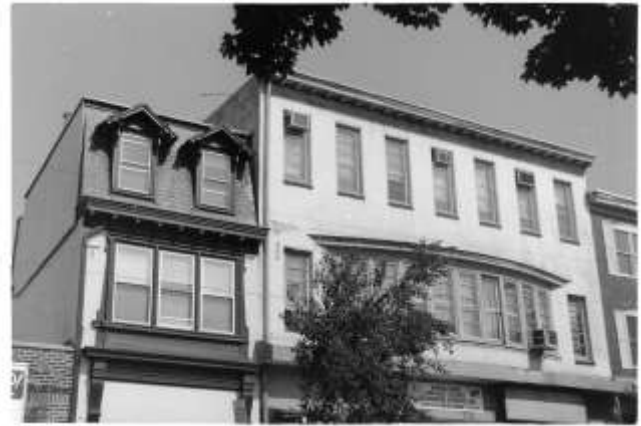
This Norristown building (center) housed Burgess’ penultimate shop. The street-level shops have been modernized, but Burgess may have peered down from the bay window.
